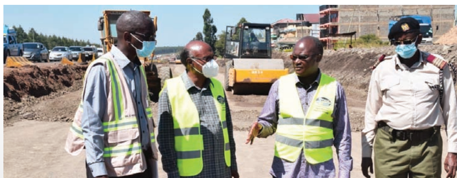
Transport CS James Macharia (second right) inspecting the ongoing construction of the 84Km Kenol-Sagana-Marua Road.
