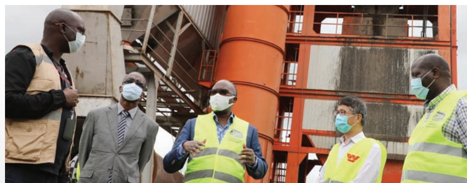
Transport CS James Macharia (centre) inspecting the initial construction of road expansion works of the 84Km Kenol - Sagana - Marua Highway into a four-lane dual carriageway way.
